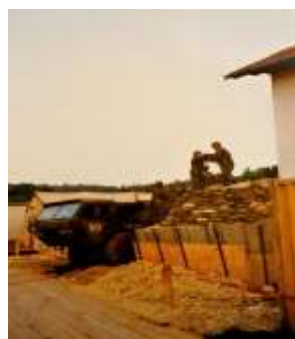
14,000 filled bags and placed!
